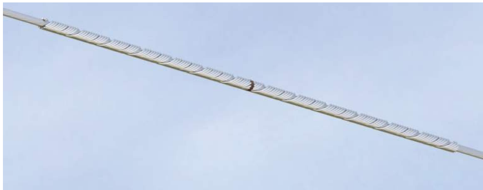
Repair Rods Installed on OPGW
